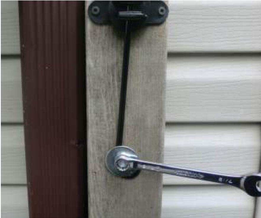
Using a wrench fix the hoop to the post/tree with the lag bolt and large washer. Ensure that the hoops point inwards.
