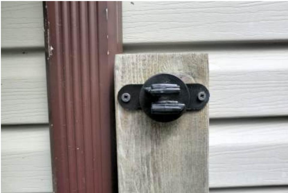
Screw the plastic clip onto the post near the top. Drill a pilot hole 6 inches lower down.
